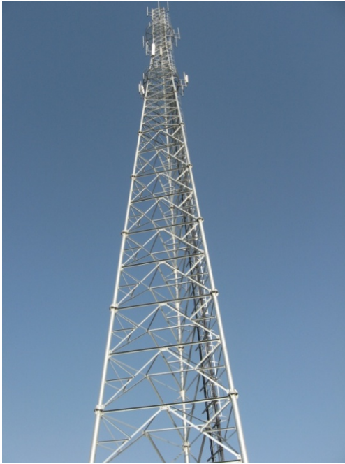
BS mast: Framework of angle iron
