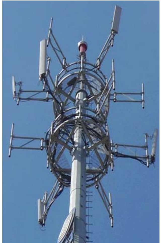
BS mast: Single-tube tower
