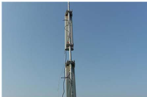
FIGURE 23 Antenna configuration for down-tilt in vertically separated antennas
