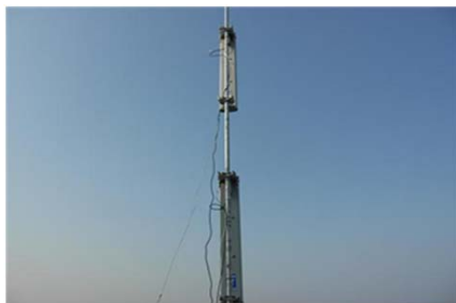
FIGURE 21 Antenna configuration for vertical separation
