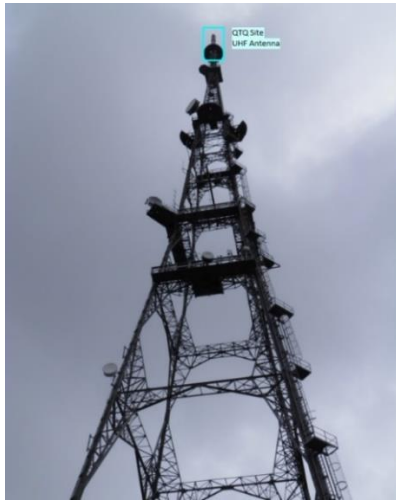
FIGURE 3-19 Mt Coot-tha Q-Site Tower
