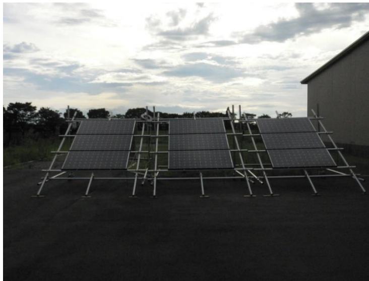
FIGURE A1-1 Examinations with actual equipment
