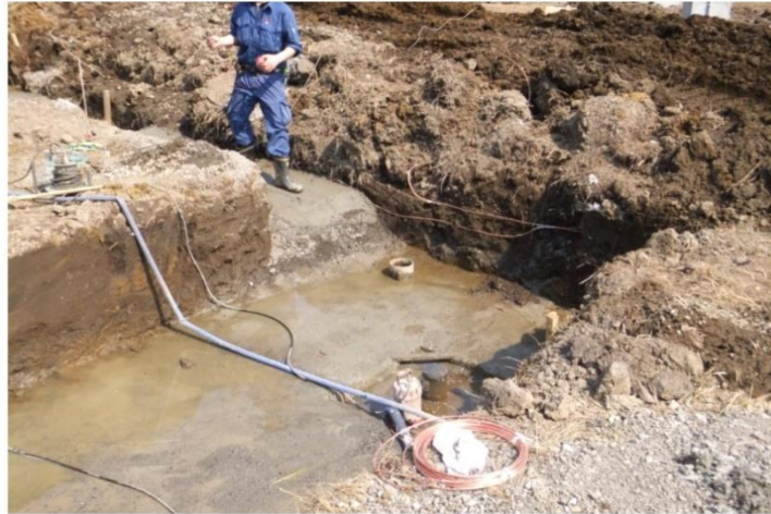
FIGURE 8 Connection to the existing grounding radials
