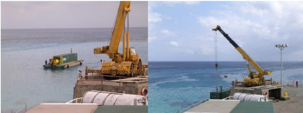
FIGURE 19 Offloading at Ascension Island
