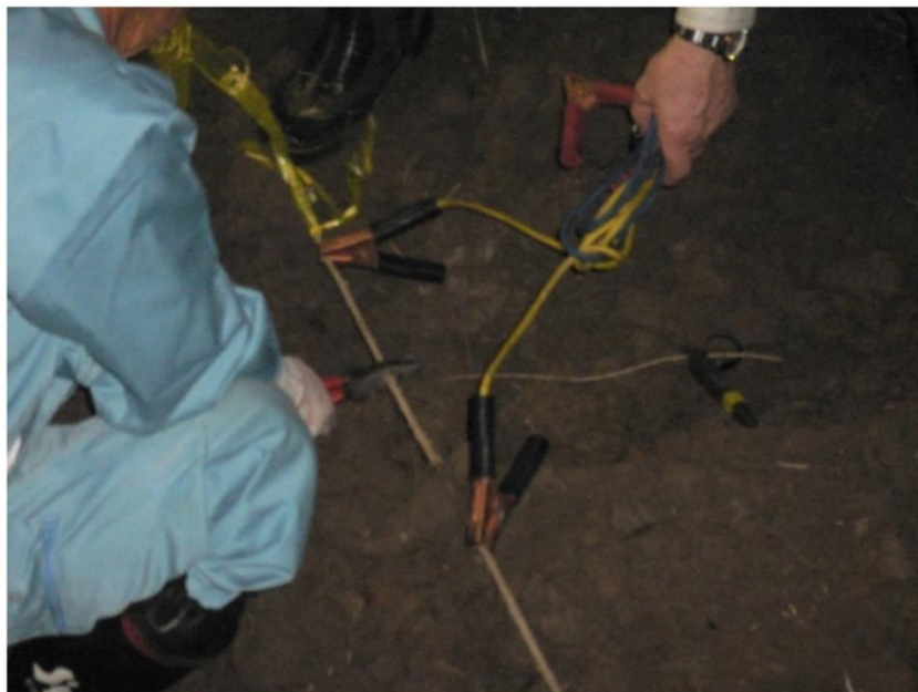
FIGURE 5 Cutting off grounding radials
