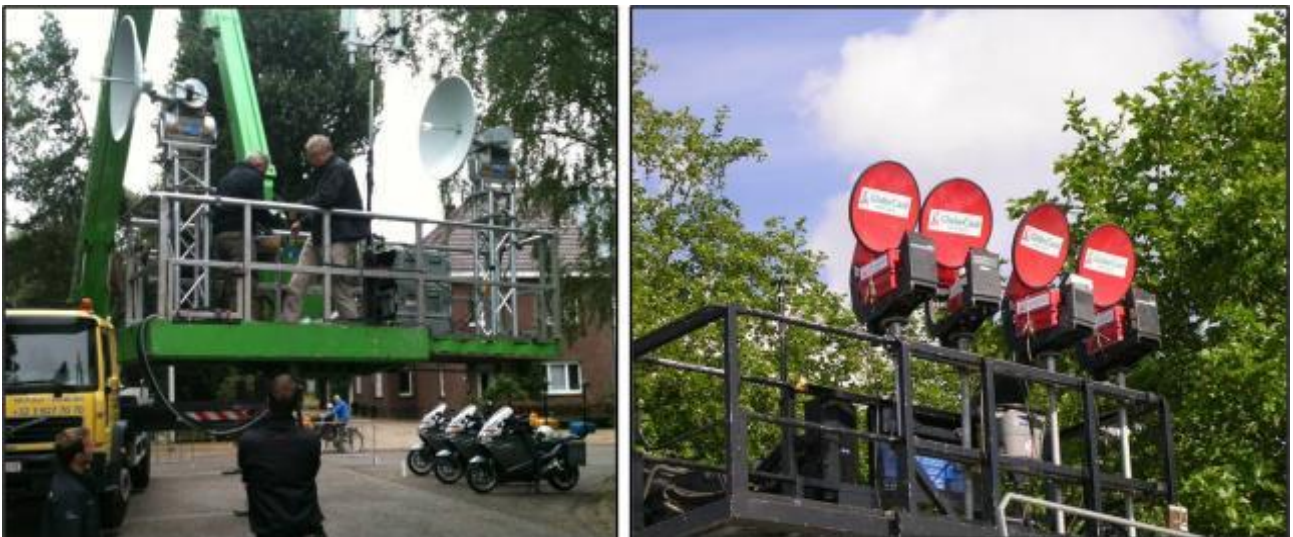
FIGURE 15 Temporary point-to-point video links
