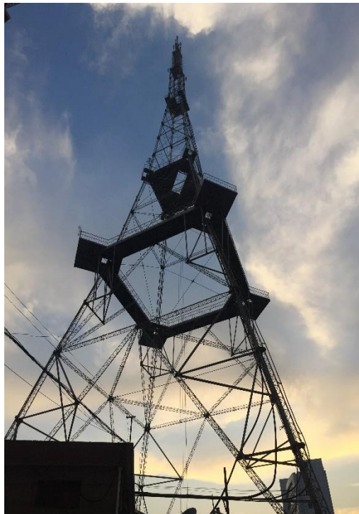
Transmission station antenna
