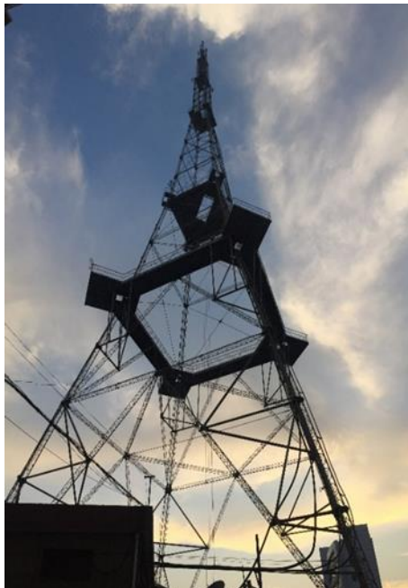
Transmission station antenna
