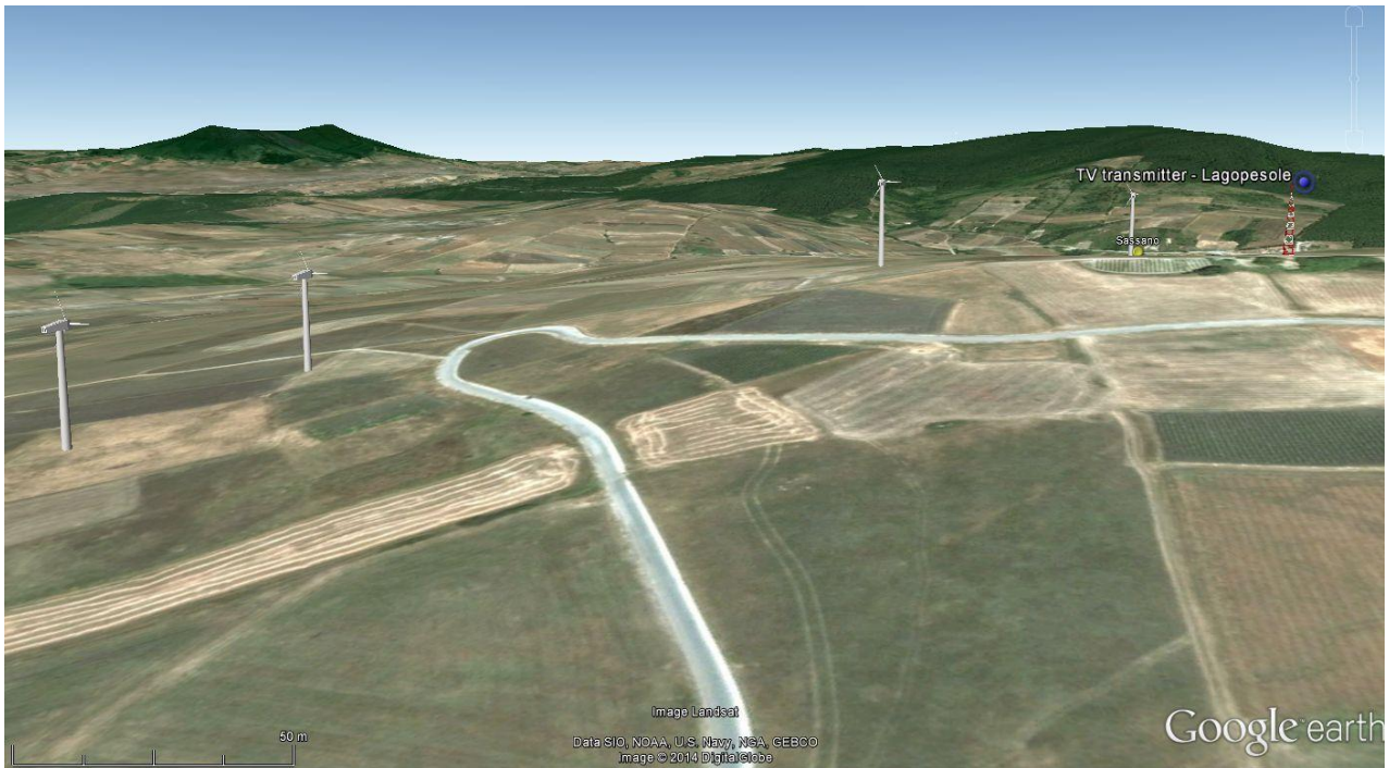
Aerial view of the wind farm and Lagopesole transmitter station
