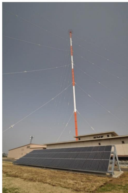
FIGURE 3 12 kW solar power generating facility
