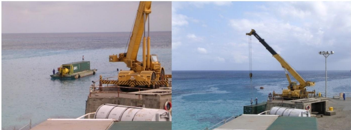
FIGURE 19 Offloading at Ascension Island
