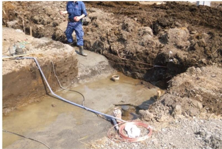
FIGURE 8 Connection to the existing grounding radials
