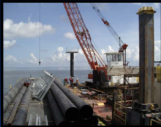
Hardened tide gauge on Gulf of Mexico coast after hurricane Katrina
