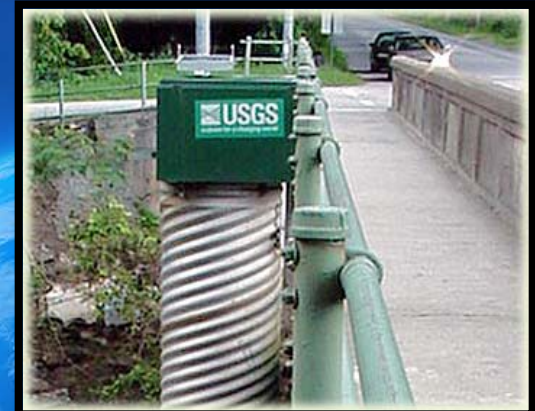
Stream gauge mounted on bridge
