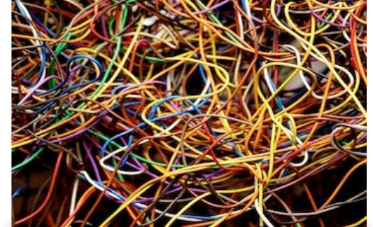
No network control
