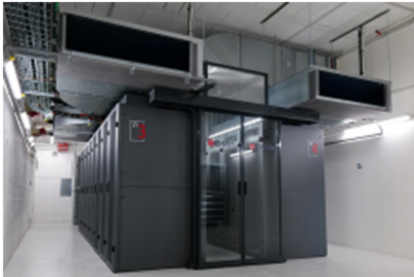
Figure 5: IT room containment
