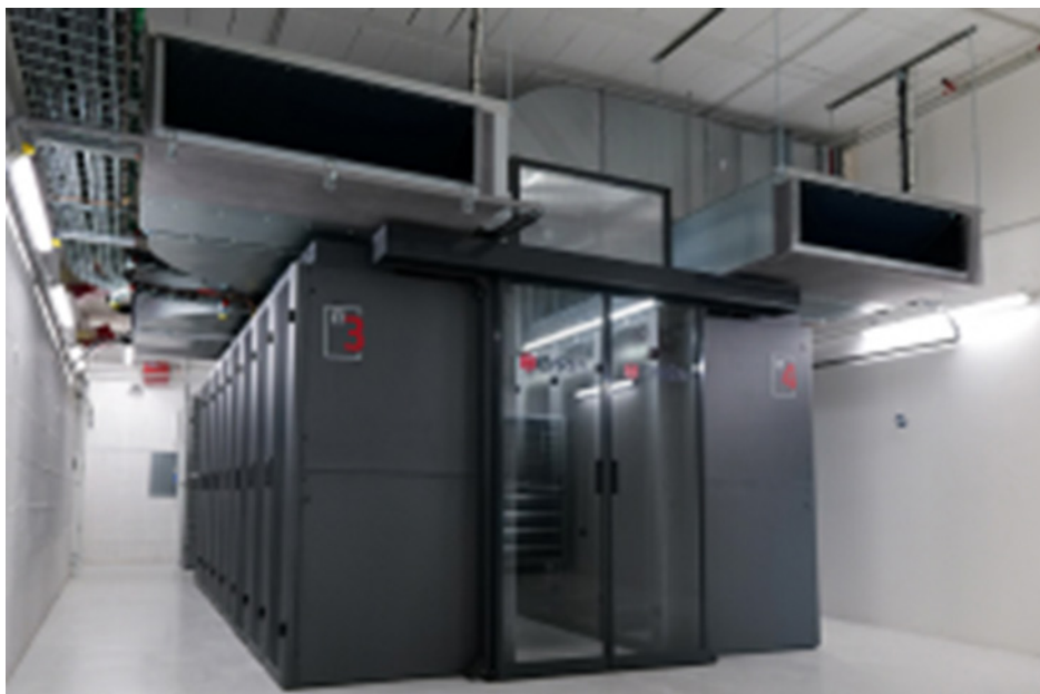
Figure 35: IT Room Containment
