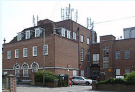
Figure 5-5: Cell site placed atop an existing building
