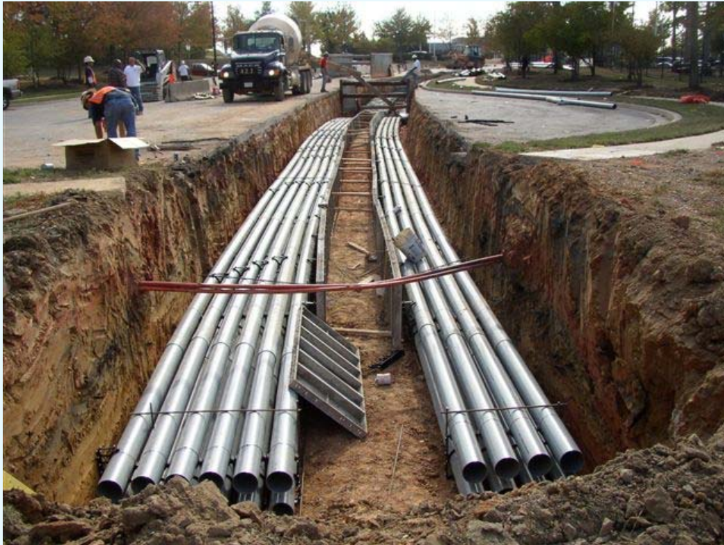
Figure 4-11: Ducts laid in a trench
