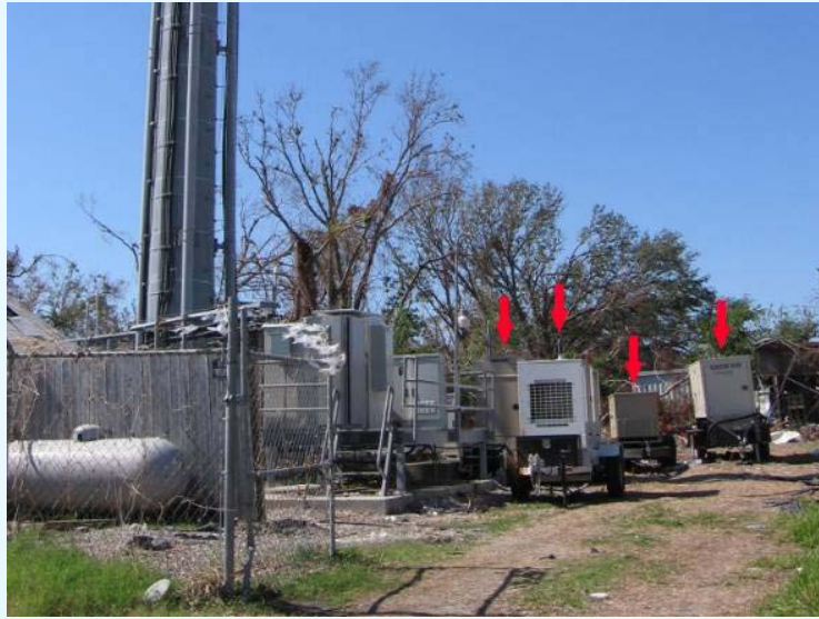
Figure 3-19: Cell site in Biloxi, MS With 4 portable gensets
