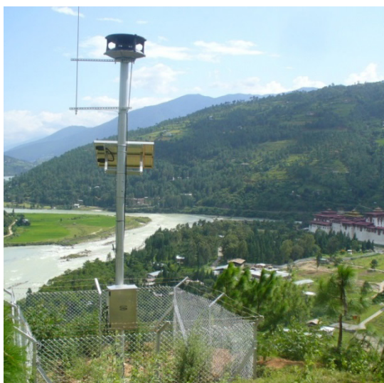
Figure 3A: GLOF Early Warning Station
