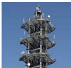
Figure A-42: Large-zone base station
