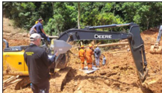
Figure A-33: Locating and digging operations in the rescue areas
