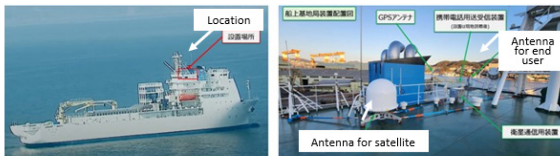
Figure A-38: Shipboard base station
