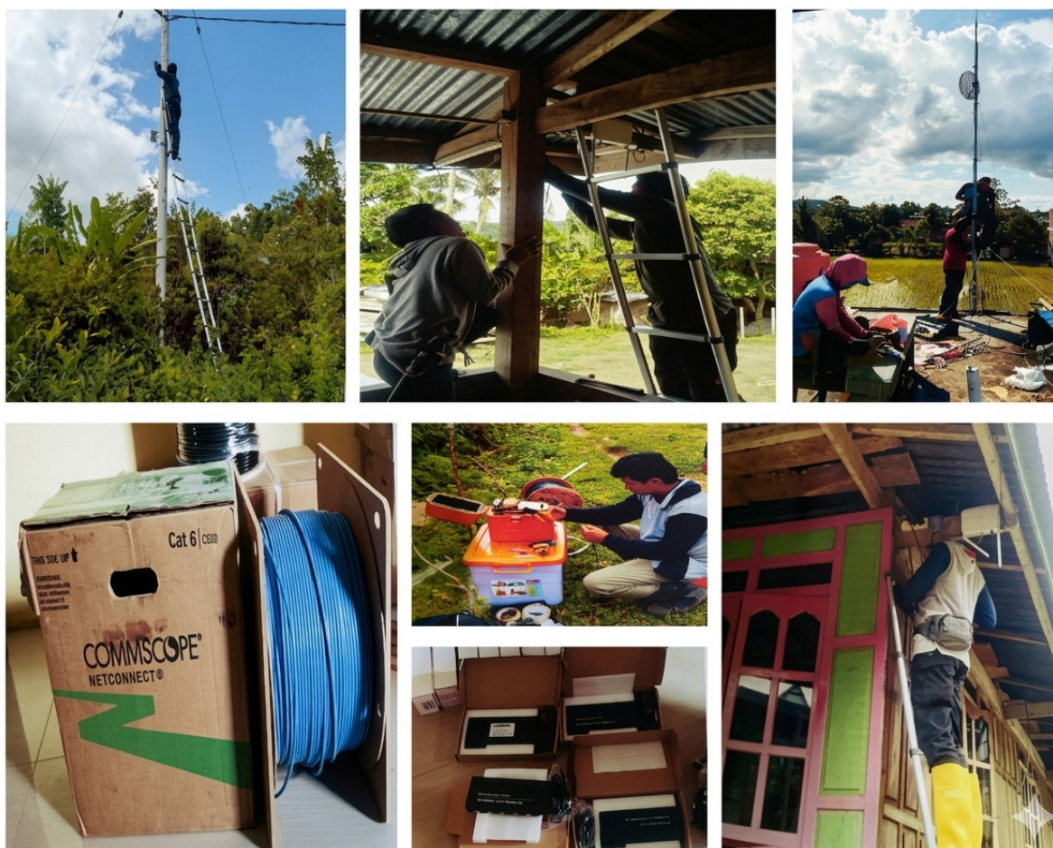
Figure 3: Technicians installing network infrastructure in Cenrana
