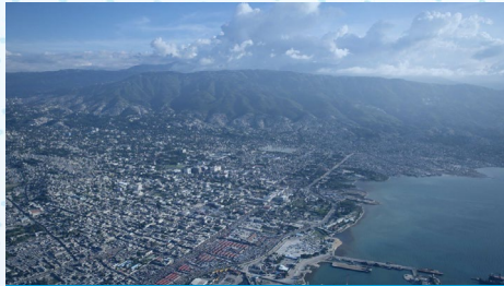
Haiti's National Emergency Telecommunications Plan
