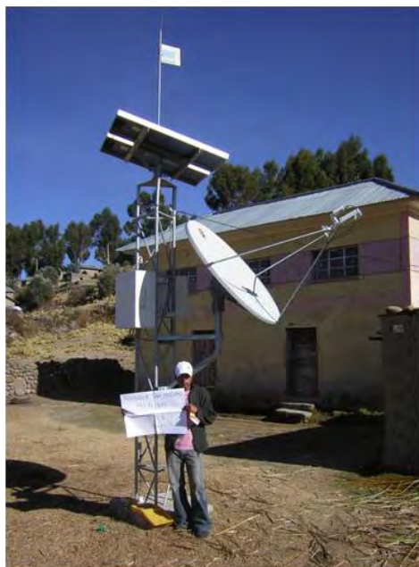
Picture N° 18: VSAT transport network infrastructure in Puno, in the Peruvian highlands
