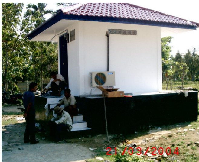
Figure-7: AGW Shelter in Madat
