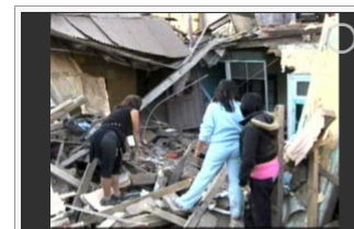
People look through the rubble of a home in Santiago Chile in this image from APTN following an earthquake early Saturday morning Feb. 27, 2010. (AP)
