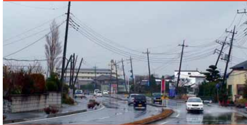
Surfacing of NTT's manhole
