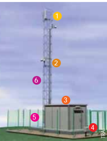
Figure 1 — Partage passif des infrastructures de services mobiles (partage de sites)
