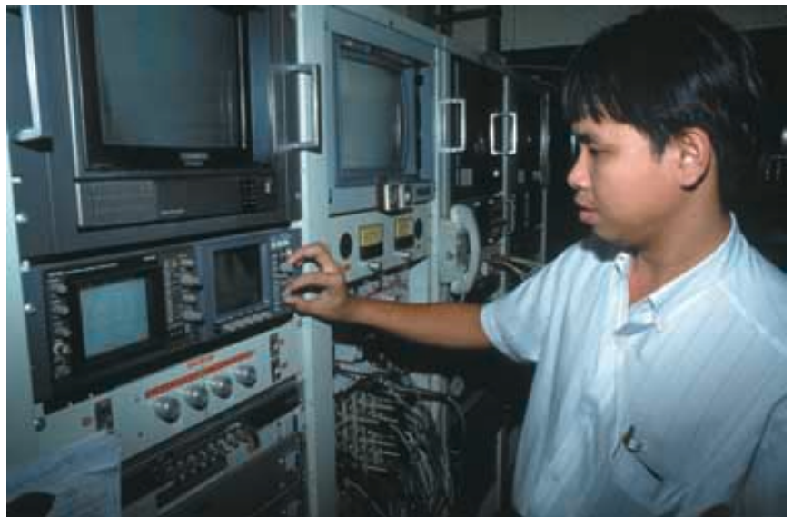
Earth station monitoring room in Bangkok
