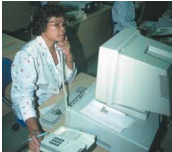
Telephone exchange in Thailand
