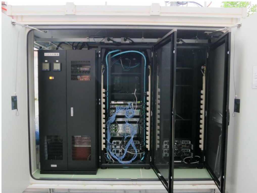
Figure 6 – Components inside the MDRU
