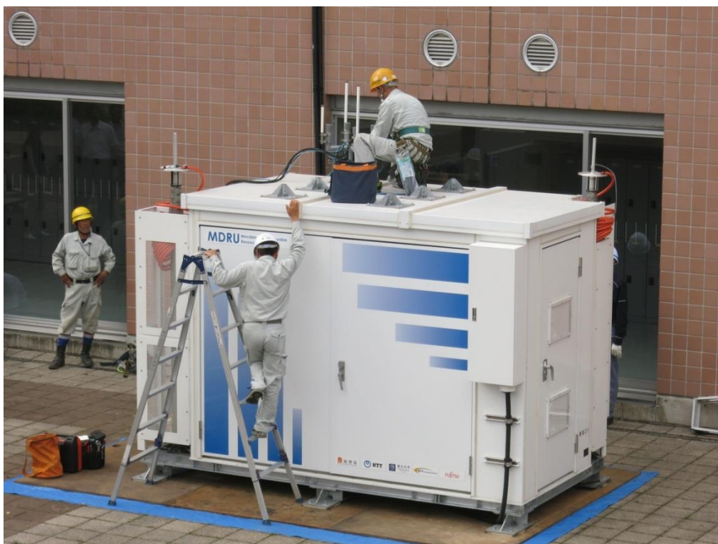
Figure 3 – Deploying and configuring the MDRU at the remote site
