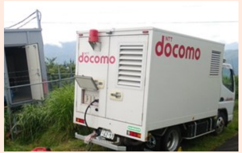
Movable power station
