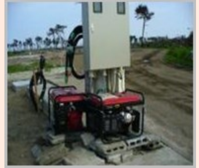
Portable power generator
