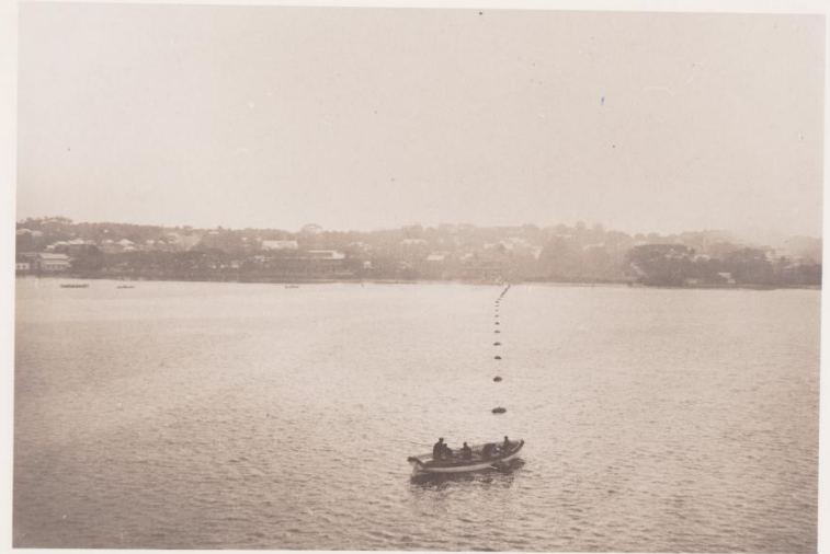
CABLE SHORE END LANDING - 1902
