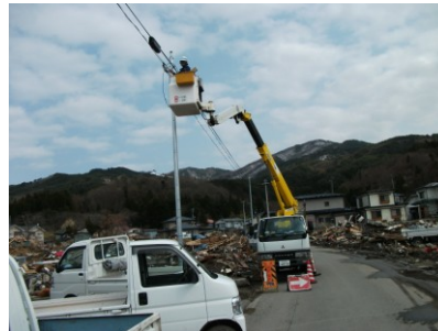
[Step 4] Connections of aerial cables
