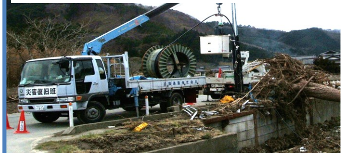
[Step 2] Installation of aerial cables
