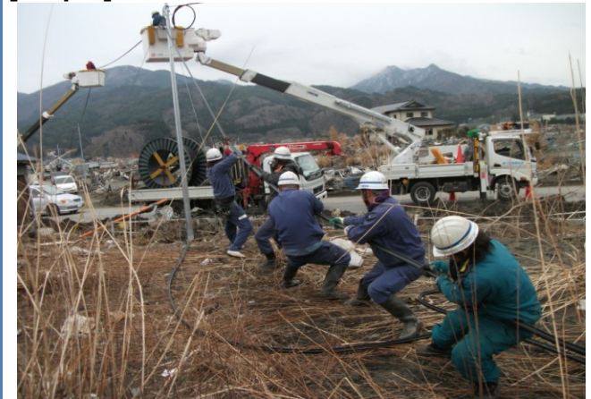
[Step 2] Installation of aerial cables
