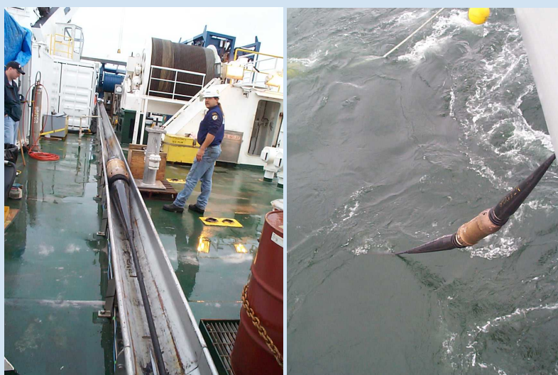
Figure 5: Optical repeaters are shown during a cable installation. System electronics and lasers are located in the copper-hued housing.
