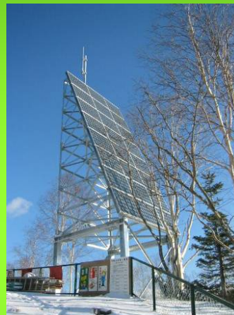
Shikotsu Lake Skyroad Mobile base station (10kW)
