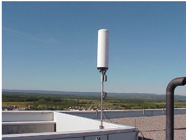
2003 Installation of 5.3/5.8 GHz Rosette Array, Ottawa
