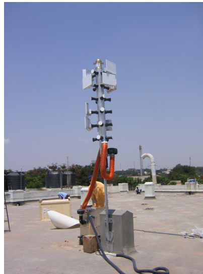
2005 Installation of 5.3/5.8GHz Rosette In Banglore,India (CDOT)
