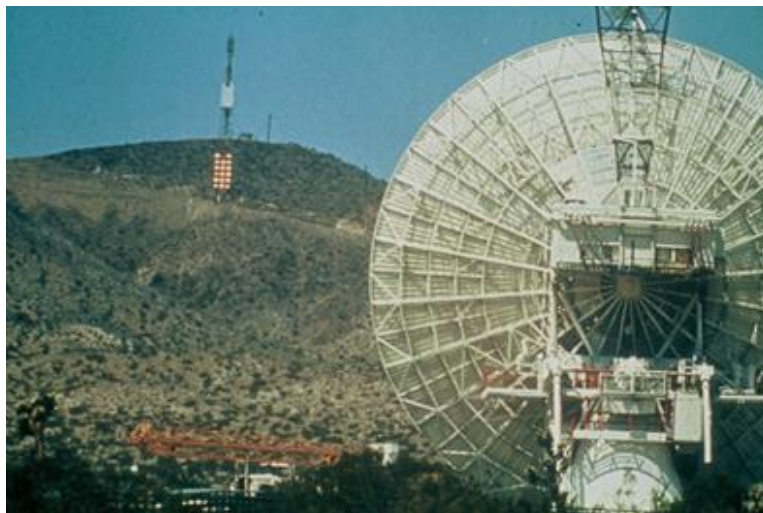
1 Mile point-to-point MPT experiment with 26 m parabolic antenna and 450kW-2.388 GHz Klystron as a transmitter and 3.4 \times 7.2 m Rectenna array as a receiver
