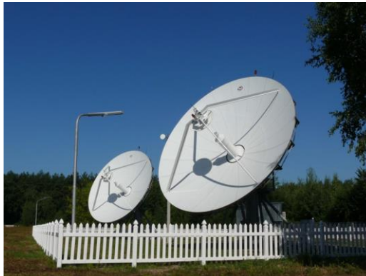
UCRF satellite monitoring station antenna system
