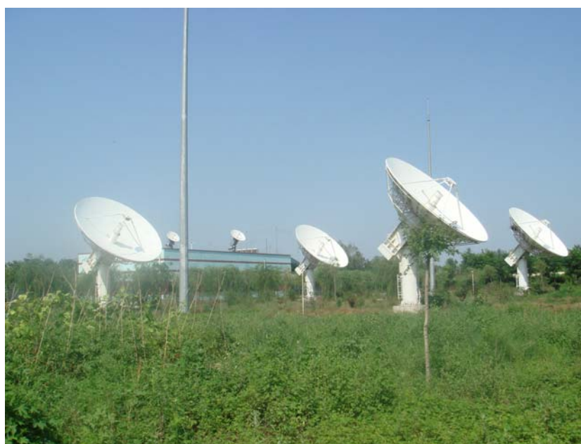
FIGURE 4 Four 7.3 m antennas belonging to System No. 2 and the reference transmitters (on rooftop)
