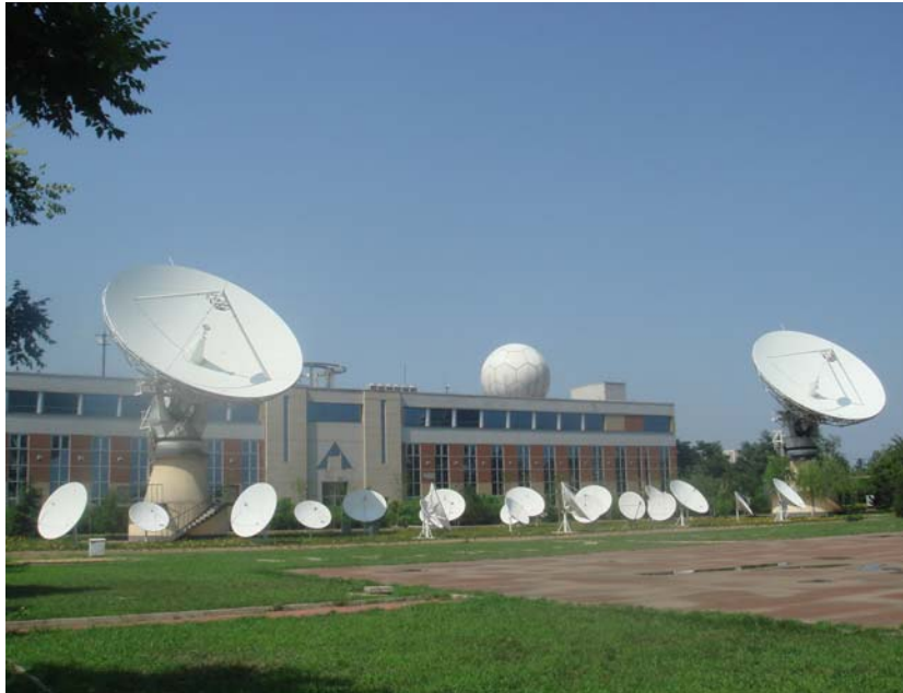
FIGURE 6 TVRO antennas for broadcast monitoring
