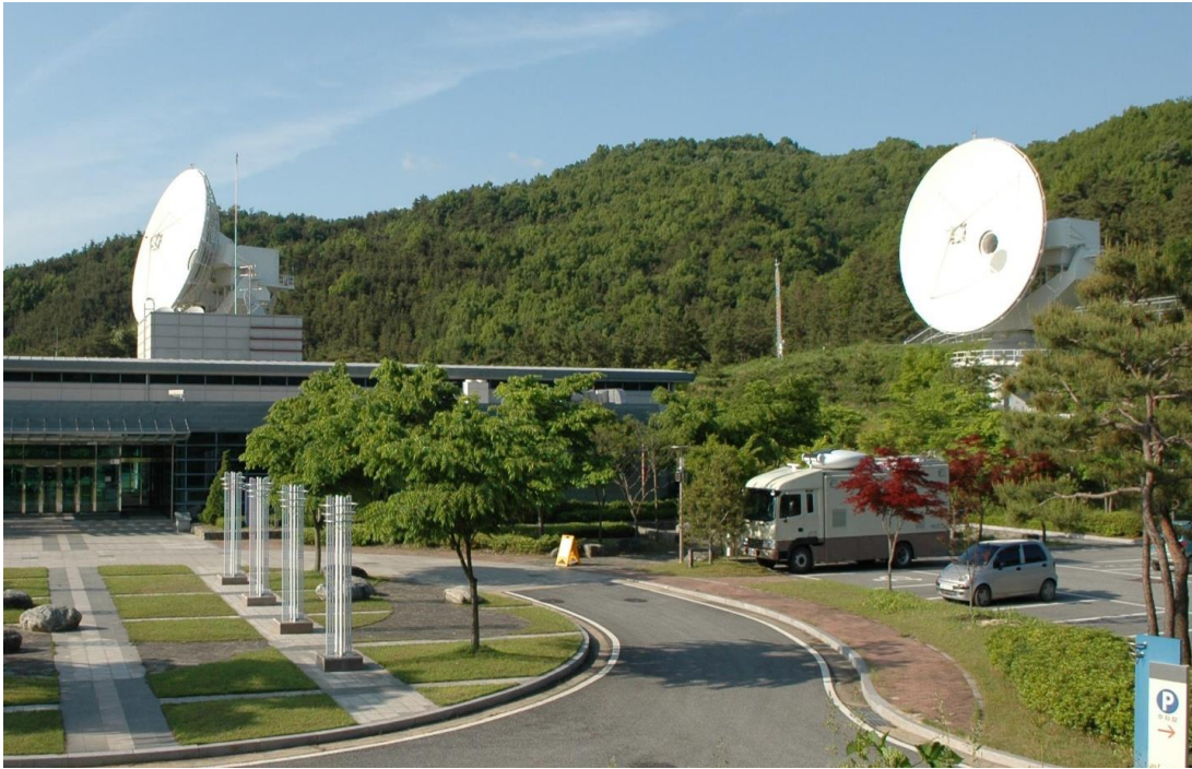
FIGURE 7 Antenna 1, 2 in SRMC
