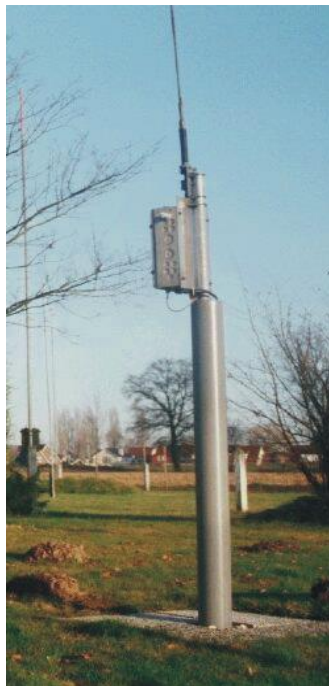
FIGURE 17 Monopole antenna
