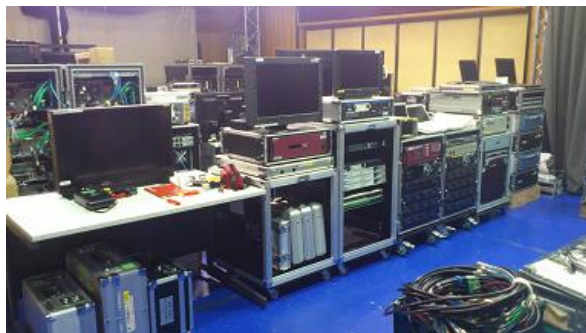
Line and transmission equipment
