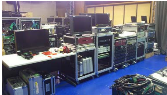
Line and transmission equipment
