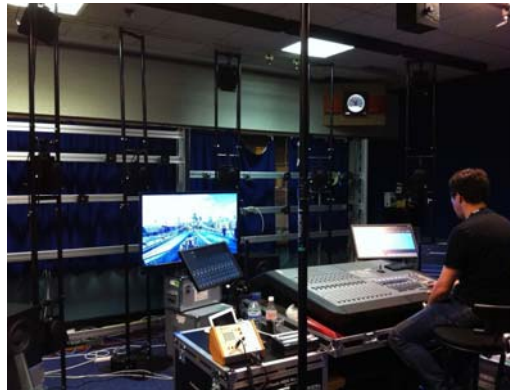
FIGURE 59 Main mixing room
