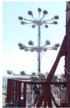
SHV camera and 22.2ch microphone array on Sapporo TV tower
