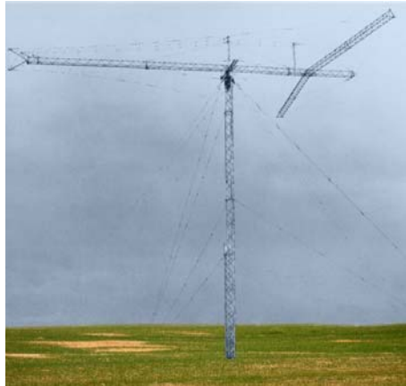
FIGURE 3-6 Example of horizontally-polarized antenna with rotator for monitoring 2 to 30 MHz
