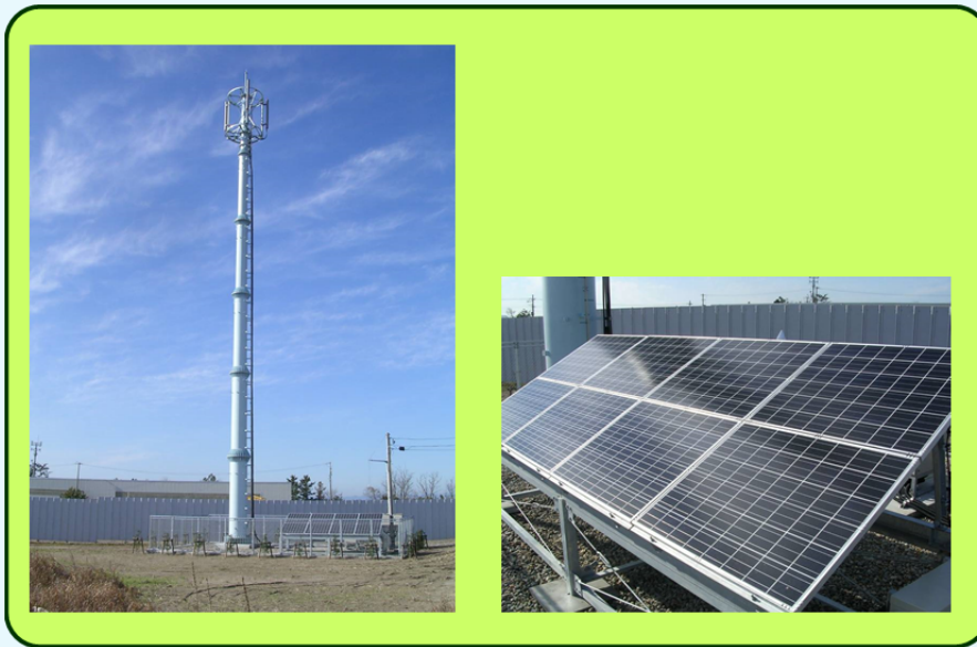
Figure 6.4 – Equipment installed for tribrid technology field trials
