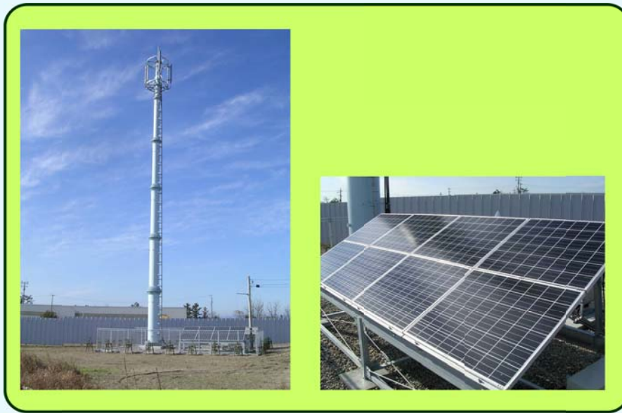
Figure 6.4 – Equipment installed for tribrid technology field trials
