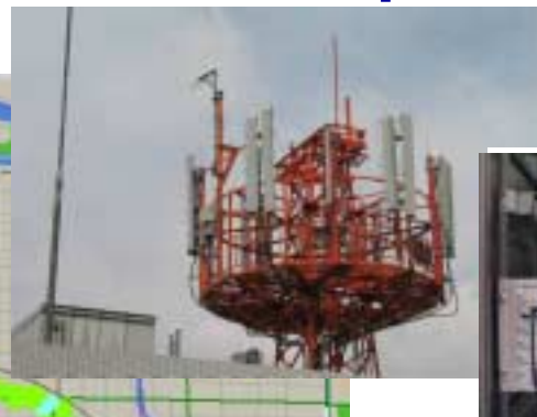
802.16e Access Point collocated with existing 3G Cellular Base Station
