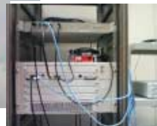
802.16e Access Point collocated with existing 3G Cellular Base Station
