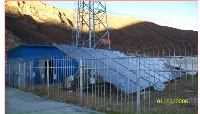
Solar/AC/DC Hybrid System
