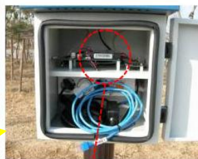
Relay for Switching Streetlight
