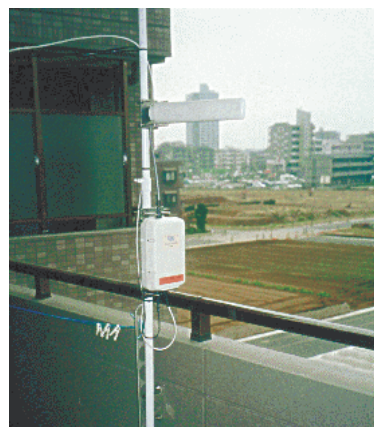
Figure 7 – Setting up an Antenna on a Veranda
